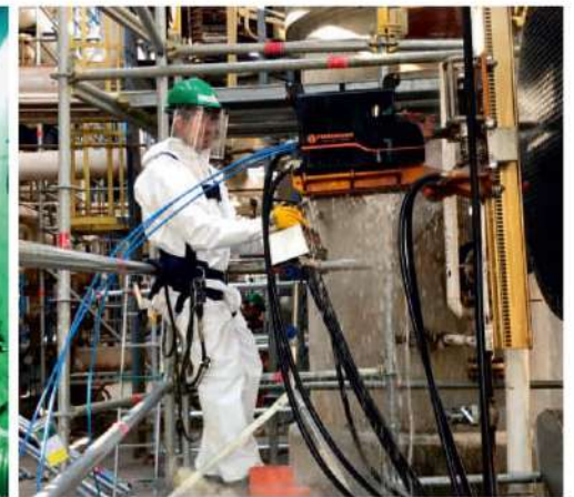
Inside and outside high pressure cleaning of bundles with proper equipment in the least possible time.
